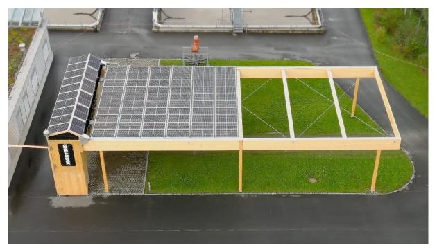
**Image 4**: Views from Urbanbox demonstration system with 6 PV module supports extended (Image: Iworks AG).
