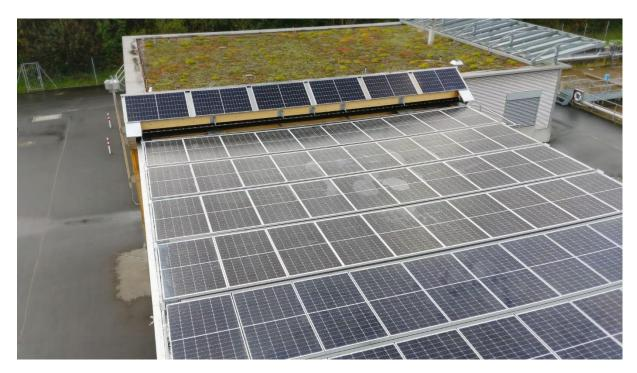
**Image 5**: Views from Urbanbox demonstration system with 6 PV module supports extended (Image: Iworks AG).
