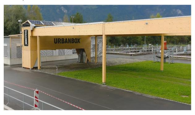
**Image 6**: Views from Urbanbox demonstration system with 6 PV module supports extended (Image: Iworks AG).
