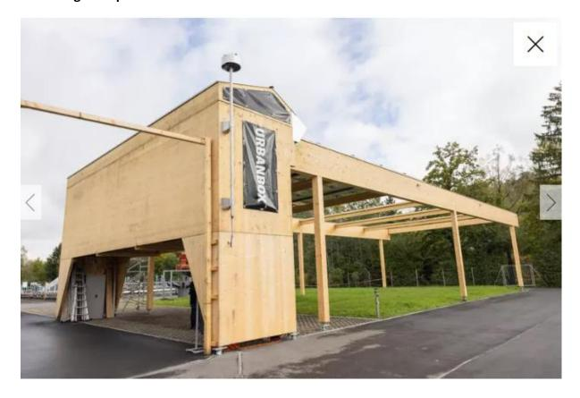
With a retractable photovoltaic roof over sewage treatment plants, parking lots or roads to produce electricity: That's the idea behind the Urbanbox. Yesterday of the lightweight photovoltaic system at the ARA wastewater treatment plant in Bendern.
